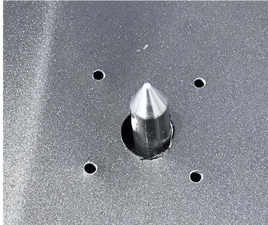
9. Use a small drill bit to make pilot holes for the hood bezel screws.
